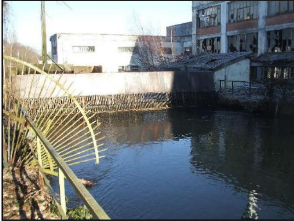
Alimentation turbine BTT
